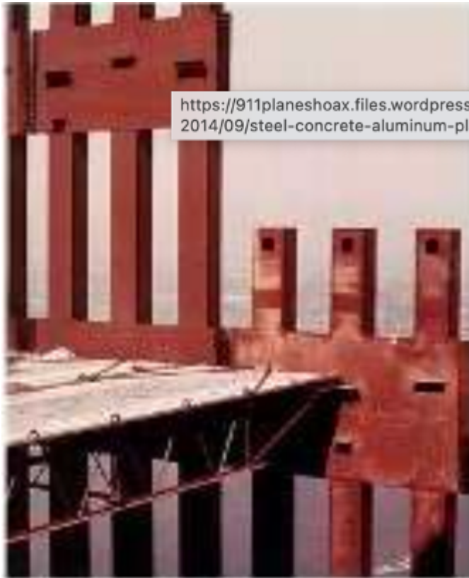
Photo during the construction of the twin towers - steel structure of the outer shell.
